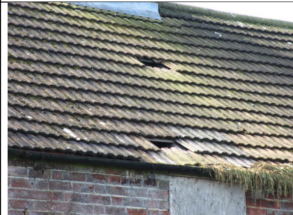
Photo 9: Missing pantiles on workers cottages
