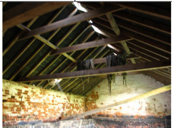
Photo 6: Inside the south side of the old barn
