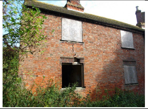
Photo 8: Open Window on south-west side of workers cottages
